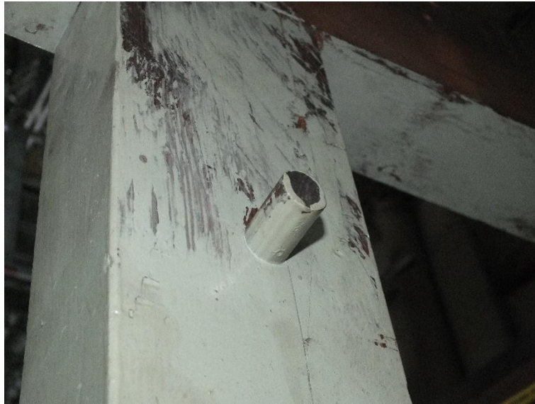
Locating dowel likely to have been for Grand Orgue rollerboard
