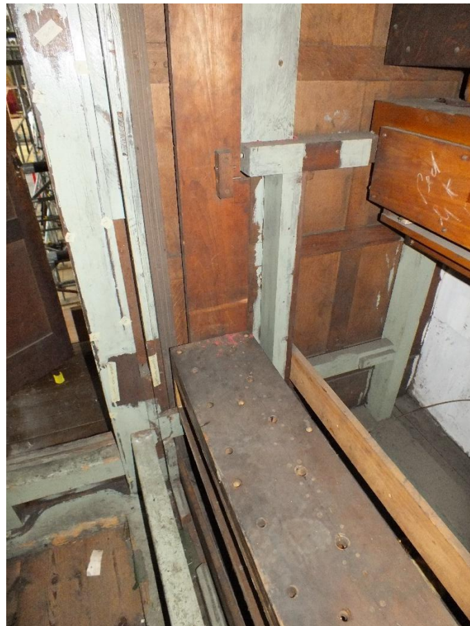
Remnants of frame for side panelling of staircase
