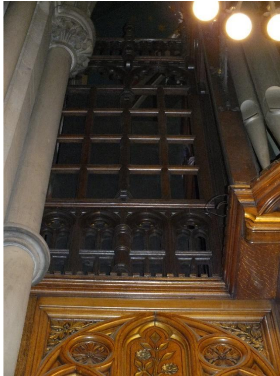
Hatching infill of 1893 at side of casework Originally the only material between the lower and upper fretworks
