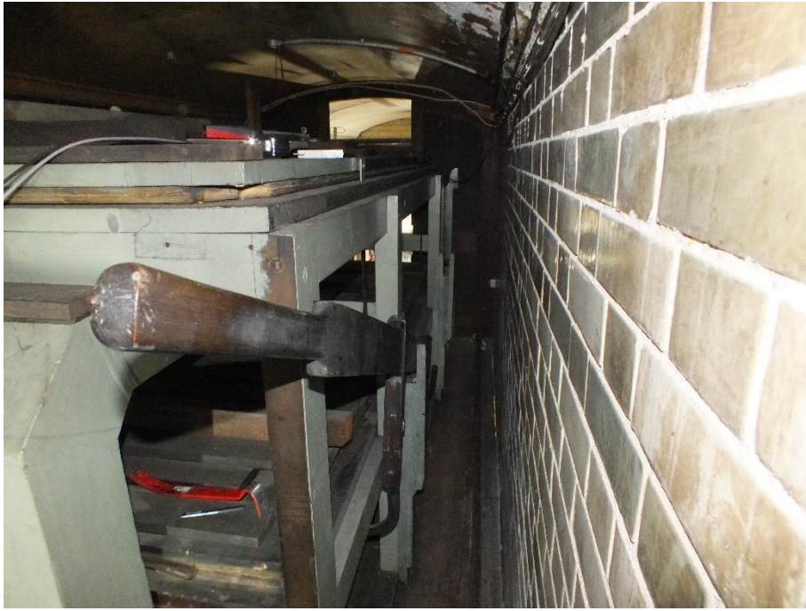
The 'accessible' of the two pumping handles in the chambre de la soufflerie
