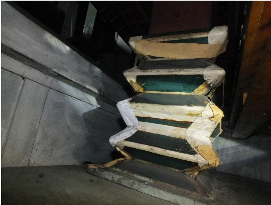
Typical condition of concertina trunks prior to dismantling
