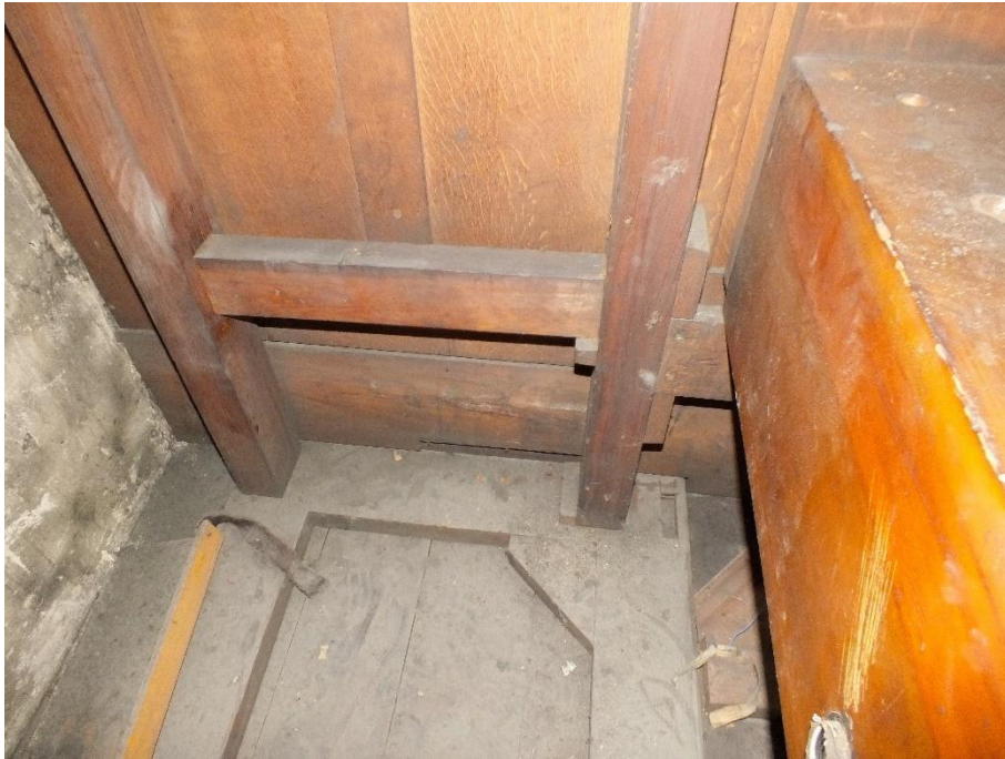
Altered 1893 Cavallé-Coll building frame for the Soubasse 32' / Bourdon 16' C chest
