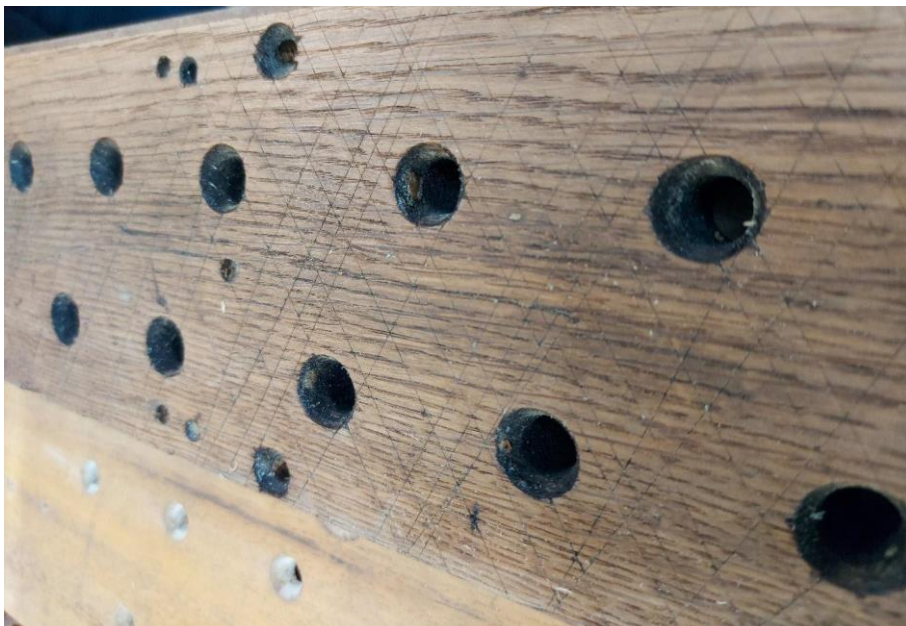
Scoring evident for glue keying Also clear that all holes chamfered for pipe feet
