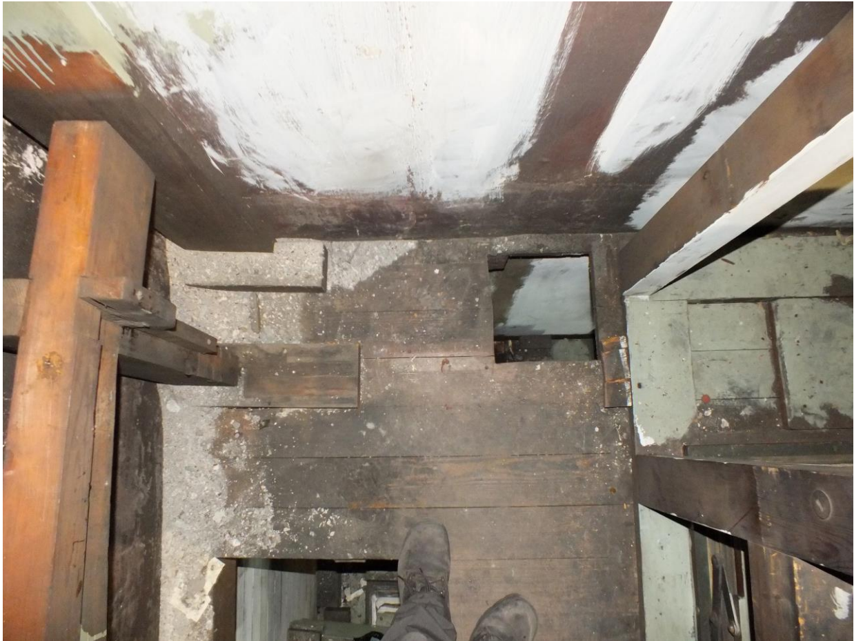
Pédale C#-side building frame (left), Positif building frame (right) as photographed from above The vertical post on the left (shortened by approx. 40cm) is let into a piece of ground frame which originally would have linked the Pédale ground frame to the Positif ground frame (a sawn-off piece can still be seen on the right)
